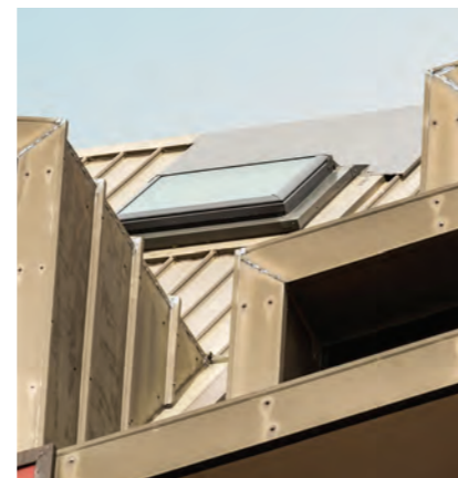
THE VELUX SKYLIGHTS LOOK GOOD FROM THE OUTSIDE AS WELL.
